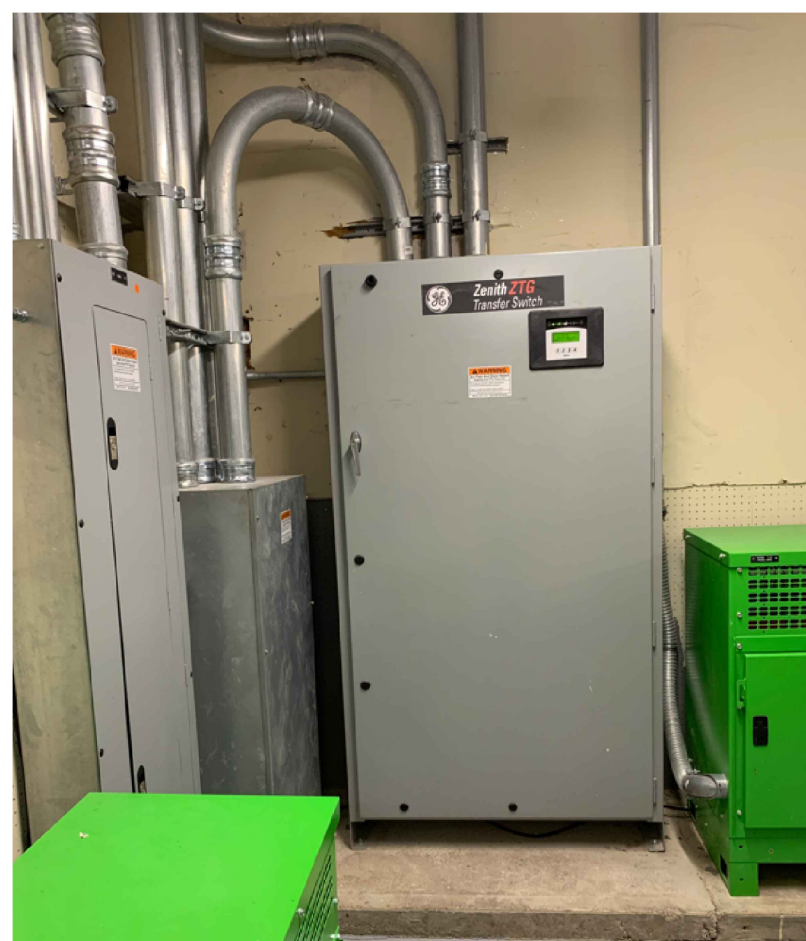
02 EXISTING AUTOMATIC TRANSFER SWITCH IMAGE SCALE: NONE
